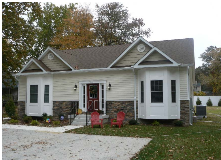
Human Services Renovations
